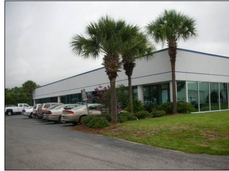
SimplexGrinnell's Orlando Office Stands Ready to Support the University of Central Florida
