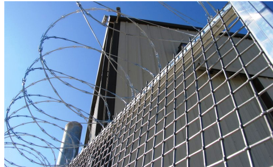
SimplexGrinnell Has Many Decades Of Experience Supporting Fire And Life Safety Systems In The Detention Market.
