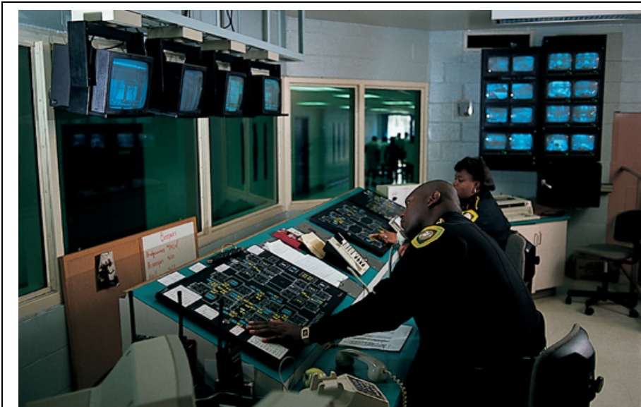
SimplexGrinnell Has Supported a Wide Range of Facilities Throughout North America
